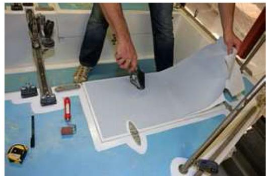
6- The laying of the anti-slip coating is finished. The maximum adhesive strength is reached after 72 hours. Nevertheless, you can immediately walk on the surface.
