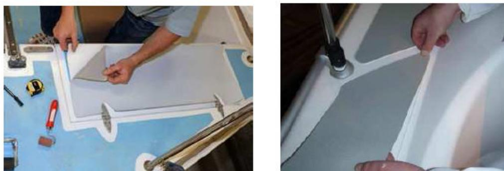
4- Unroll and peel off the protective paper, press the TBS anti-slip coating carefully and evenly with a pressure roller to avoid any air entrapment. There must be no air pockets between the covering and the substrate to prevent bubbles from forming later. Take your time with this step.
