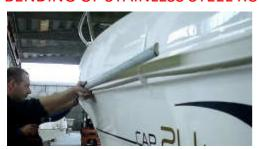
Horizontal curves with radii of <u>more than 40 cm</u> radius can be bent directly on the boat. Piece by piece should be so bent and fixed. Work your way through the radii in this way, slowly and always fixing.
