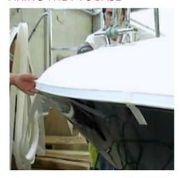
The soft base profile should be laid in one piece around your boat and fixed with vertical adhesive strips.
