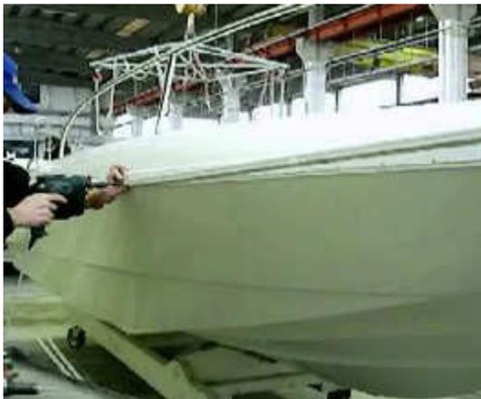
The base profile is inherently rigid but elastic to bend and is mounted “cold”. It perfectly follows the curves of the boat, even with small radii (from 8 to 10 cm - see table).
